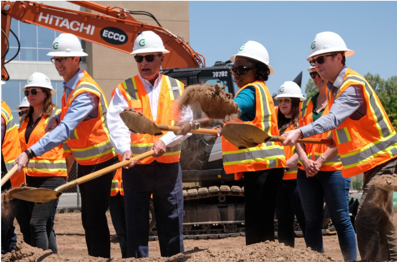
Greenlight Communities broke ground on a new apartment complex in downtown Phoenix. Katya Schwenk
